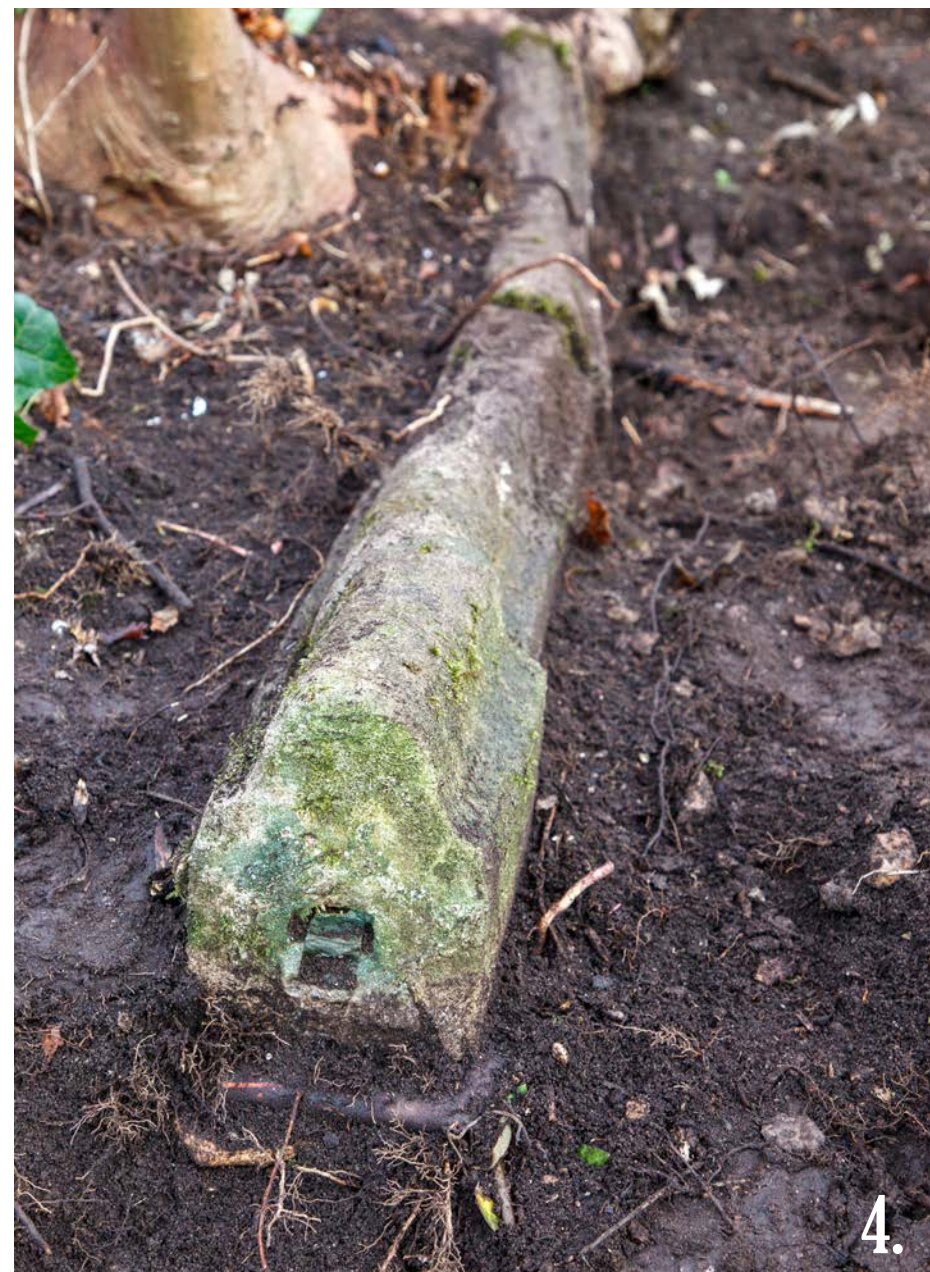
4. Detail of the end of the decorative edging along the north side of the steps, showing the curving profile and socket for the connecting plug into the next block.
