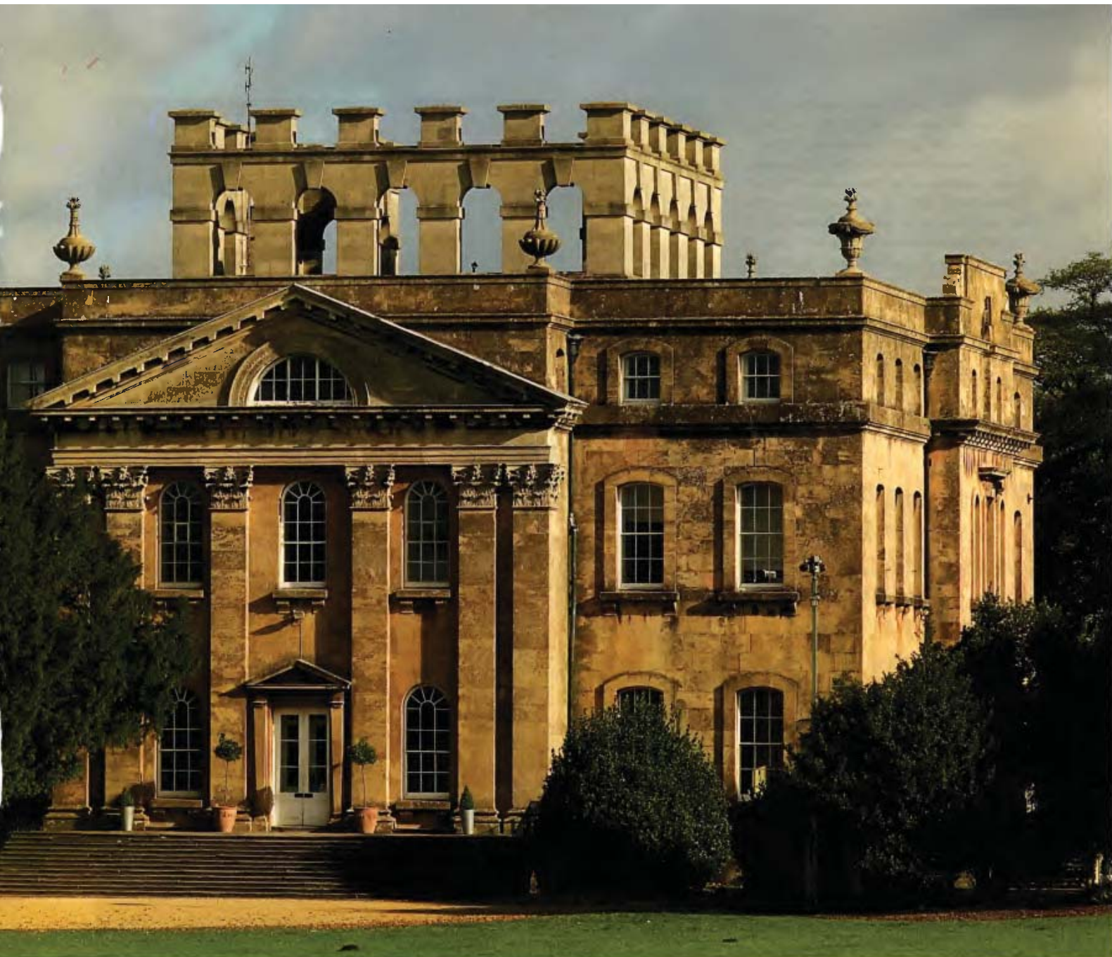
↑ Fig 2: Kings Weston House, which was designed by Vanbrugh and begun in 1711, combines the stately Palladian temple-like entrance front with a highly original skyline, which has led this house to be compared to a fantasy castle from a painting by Claude
